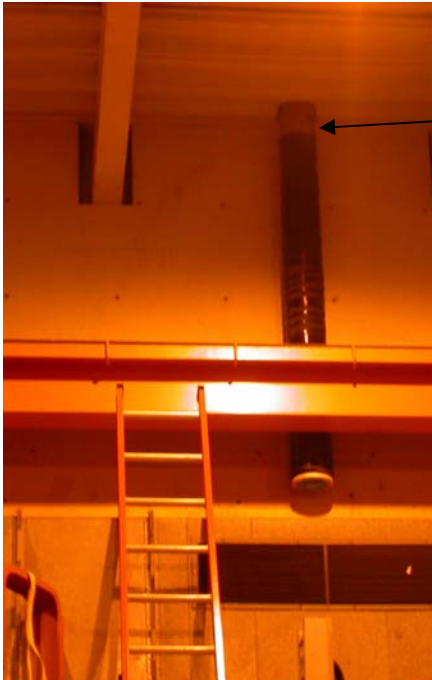
First segment of the vent line has been hung
