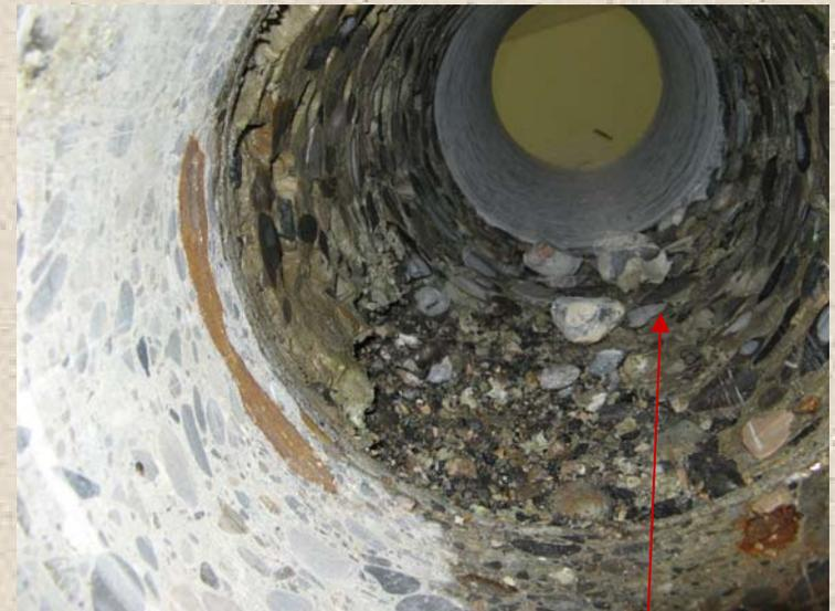
Detail of large hole – stones between the concrete walls
