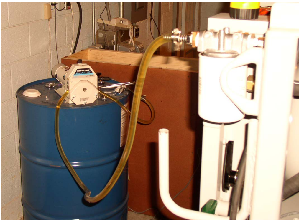
Figure IX.1: HPU Hydraulic Fluid Fill
