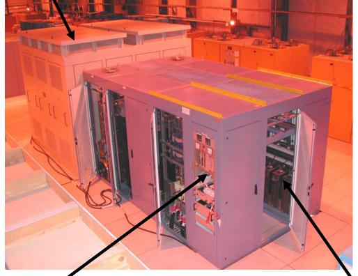
*Total DC output ratings:* 6500Adc, 950Vdc, 6.7 MW
